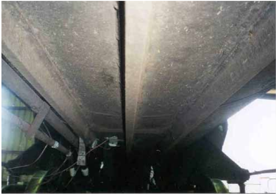
Figure 4.2 Bar-Reinforcement on Tested Railroad Tank Car
