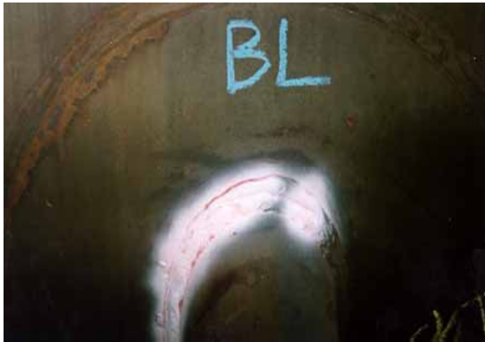
Figure 3.16 Fatigue Cracks Detected During an AE Test (Mostert 1995)
